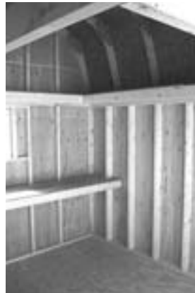
Wrap-Around Loft & Workbench
