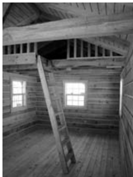
Interior with loft and ladder.
