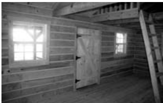
Inside of front door.
