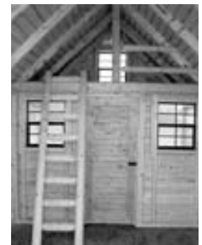
Interior of loft showing optional log railing
