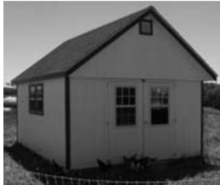
12x16' Mini-Garage, 9/12 roof pitch, vinyl doors with vented windows (used for chicken house)
